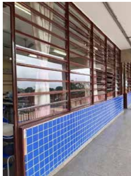
Figura 5 - Large number of windows in the classrooms providing splendid natural lighting, but significantly affecting the privacy and concentration of students. Source: Paulo Ricardo Giaquinto
